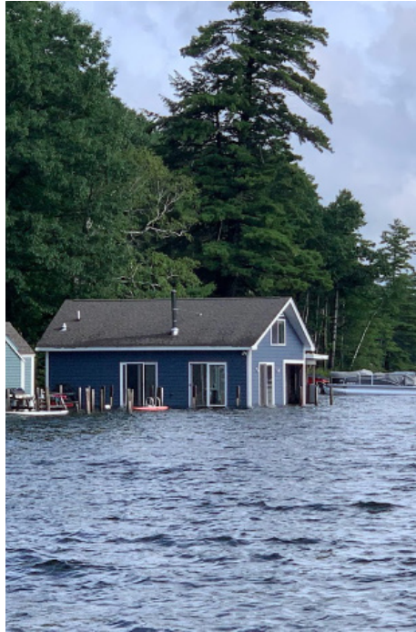
Many boat houses were inundated with water.
