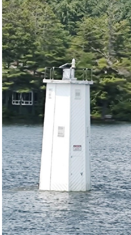
Burkehaven lighthouse under water during this summer's high rainfall.
