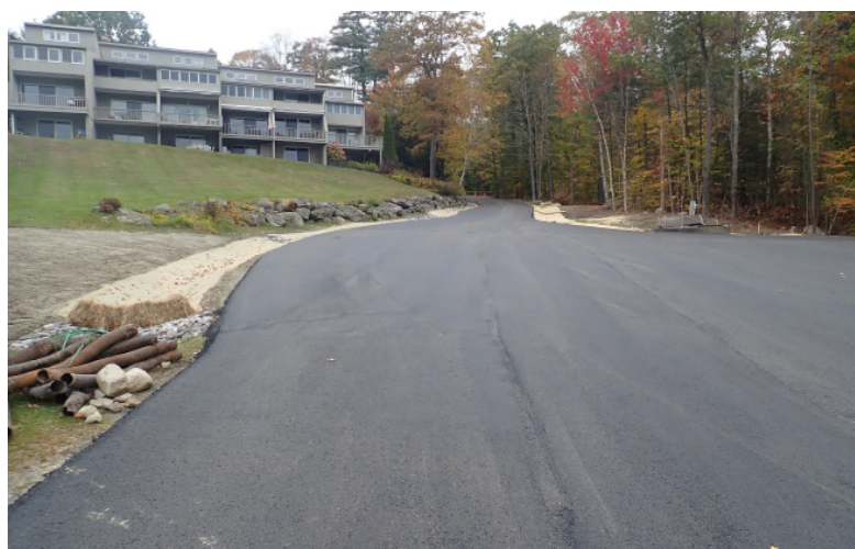
The Granliden grant site approaching completion.
