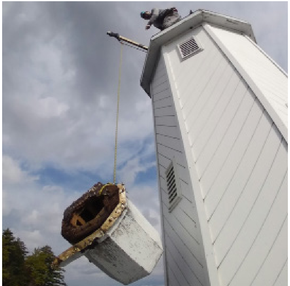
Burkehaven lighthouse roof being removed for repairs in October.
